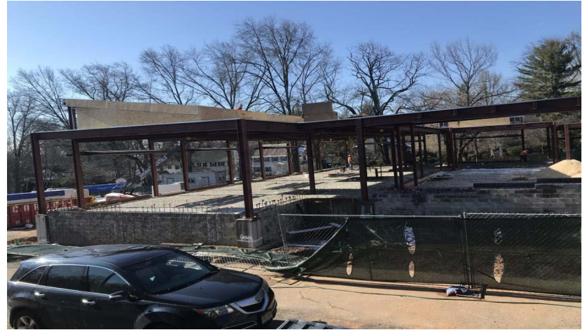
Closing metal framing and prep for SOG - Jefferson Elementary School
