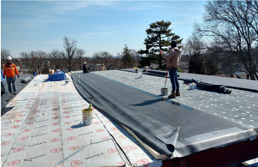
Seth Boyden School - New Addition Roof
