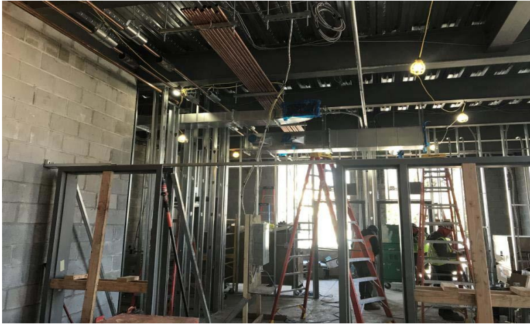
Framing, ductwork, sprinkler piping underway - Clinton Elementary School
