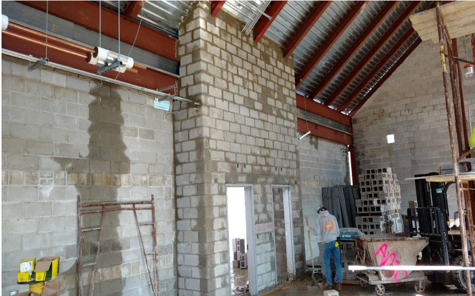
Tuscan School– Interior Classroom Entrance
